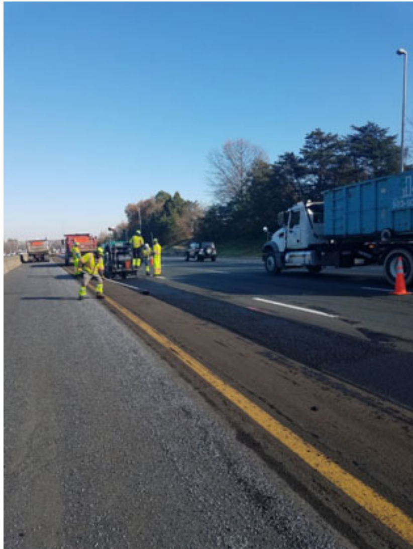
Crews working to fill potholes along I-66.
