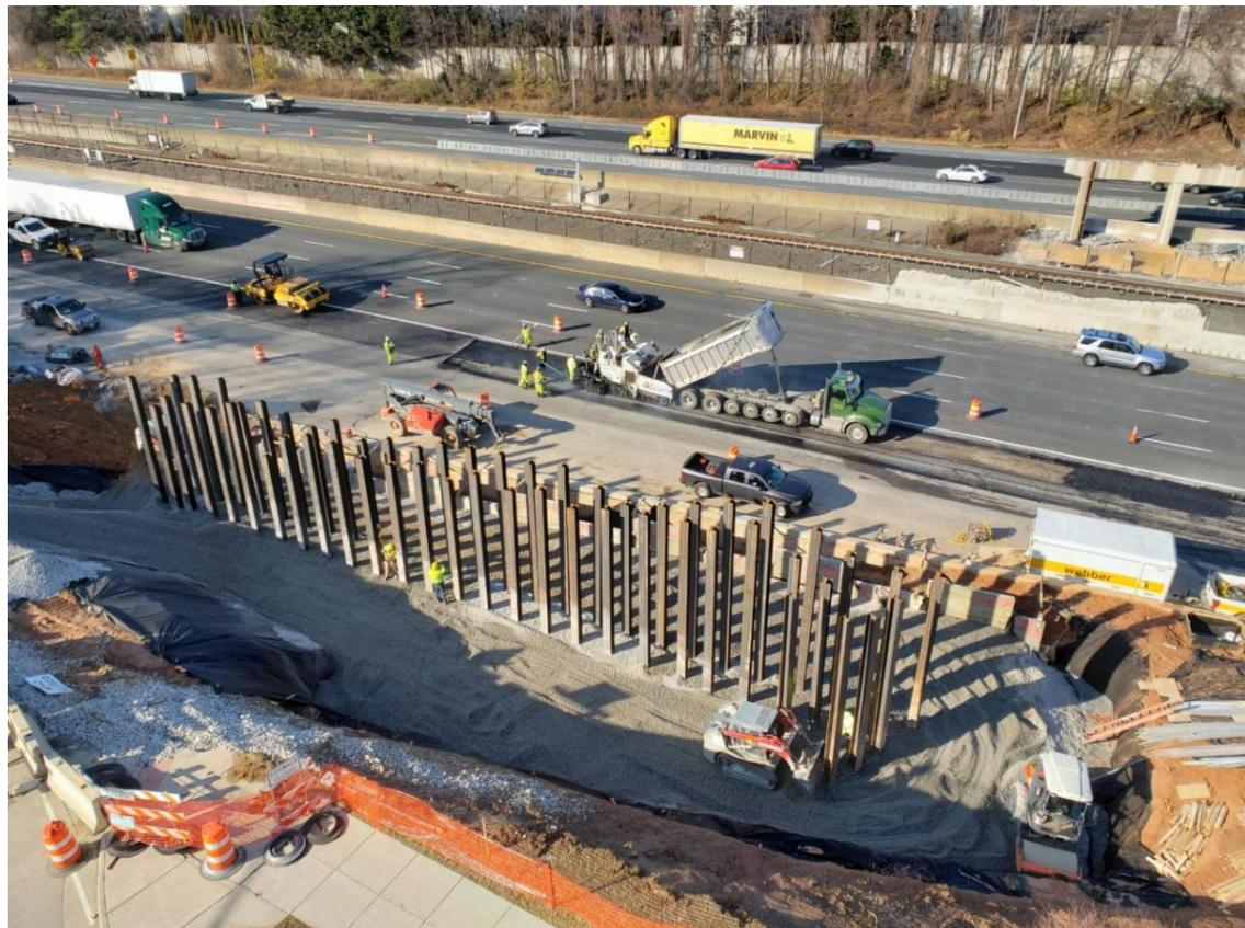
Demolition of the Vaden Drive bridge over I-66 is nearly complete. The remaining bridge piers along I-66 next to the Metrorail tracks are being demolished during overnight hours.
