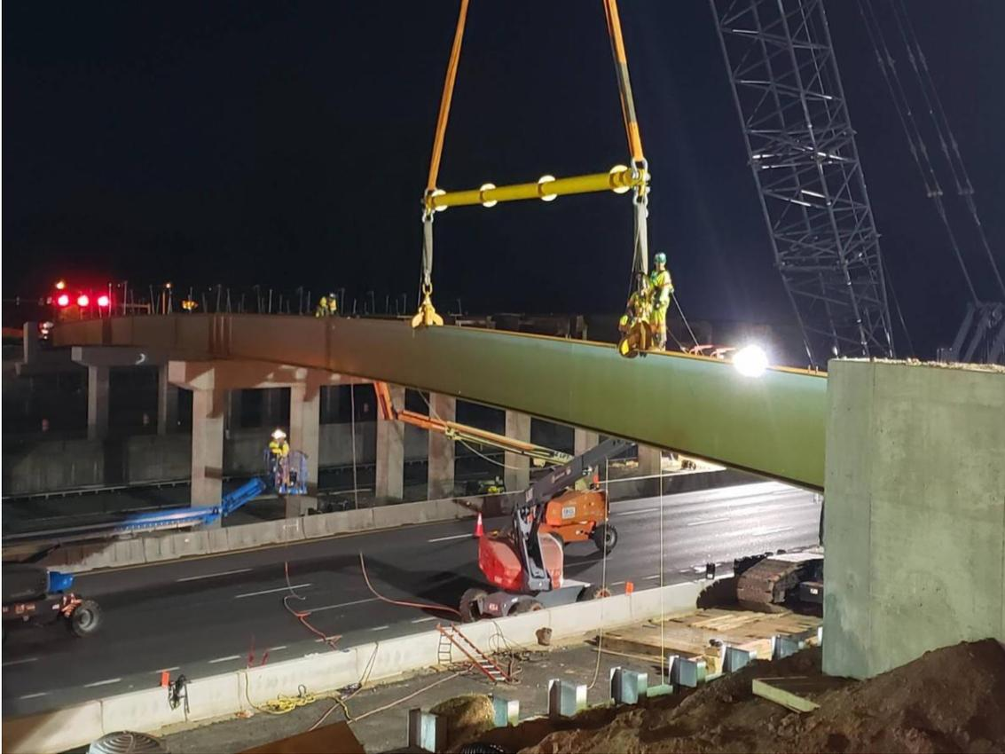
*Workers install a steel beam over I-66 West for the new Vaden Drive Bridge.*
