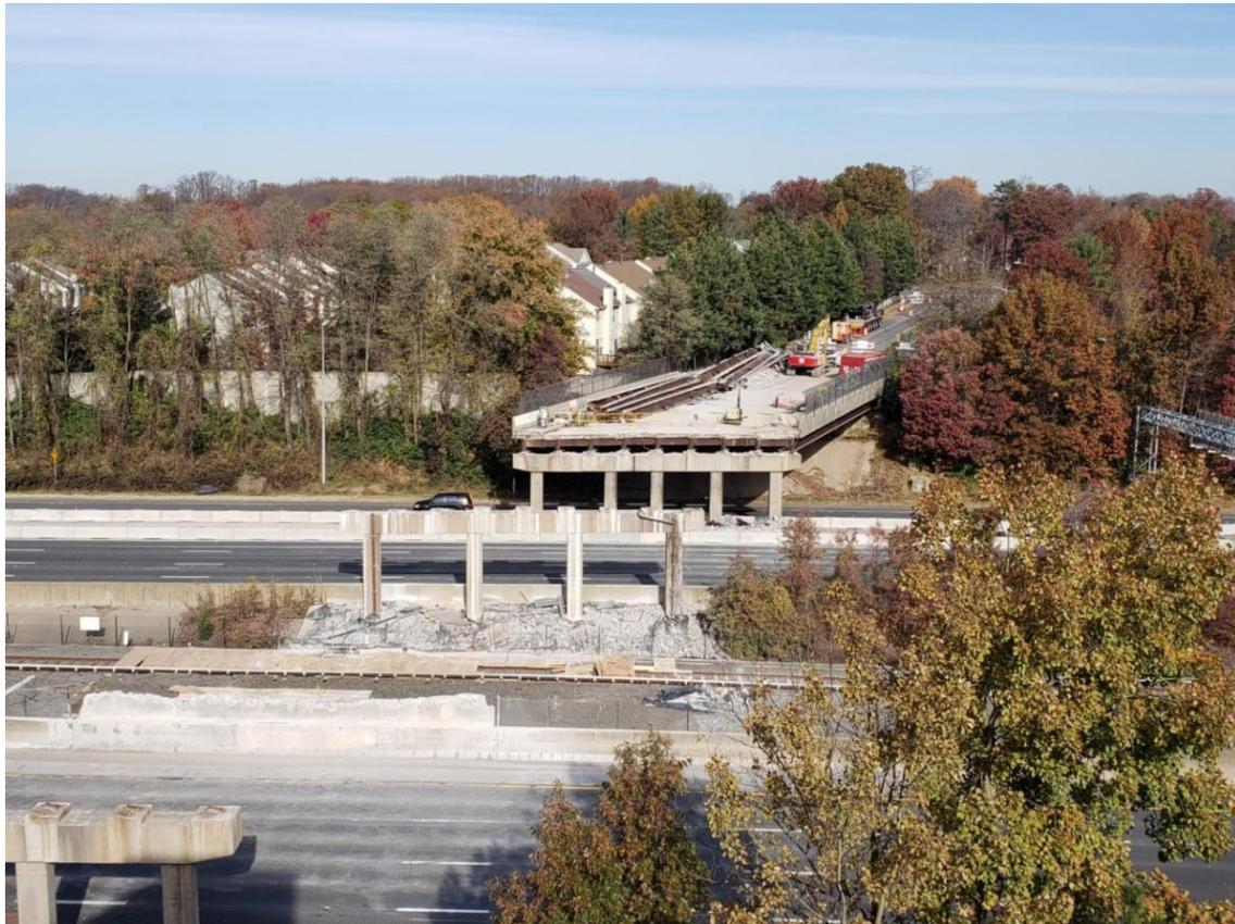
While demolition continues, construction will begin this week on the new southern bridge abutment to include pile driving during the daytime hours.
